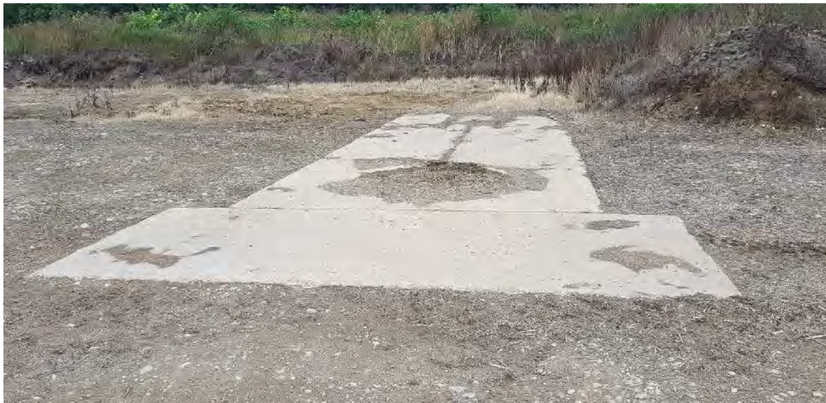
Concrete slab assumed capping decommissioned well
